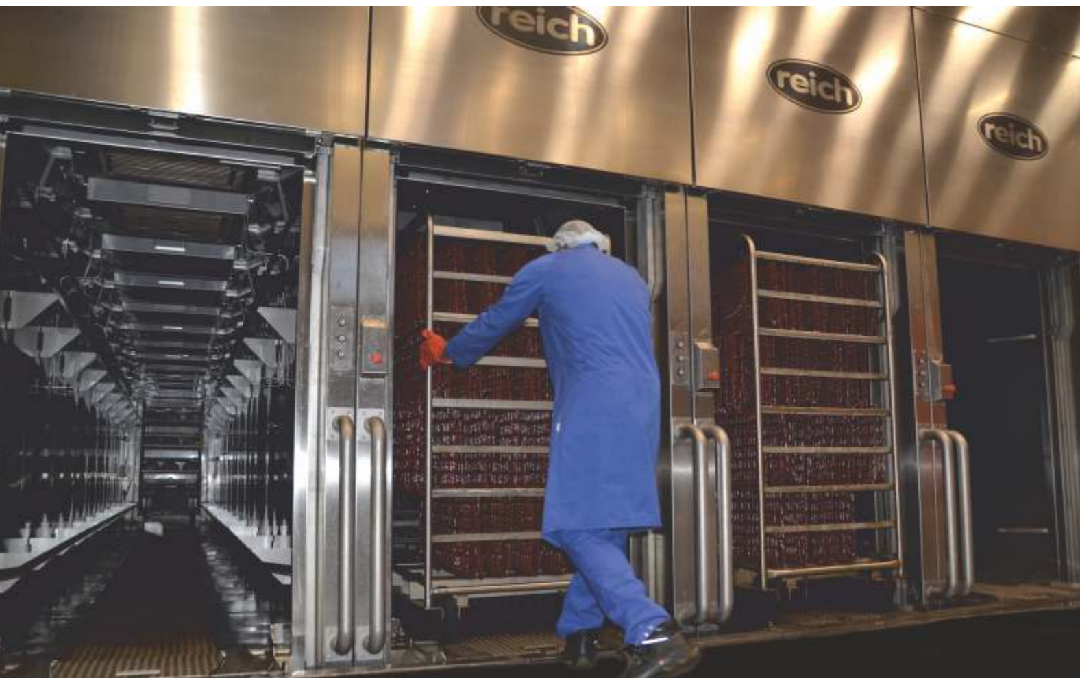
Industrial plant in the Netherlands (8 x UK 27500 BHD for 11 trolleys each with automatic lifting gates)
